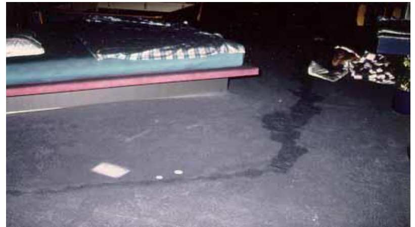
Unburned accelerator liquid on a soot covered carpet
