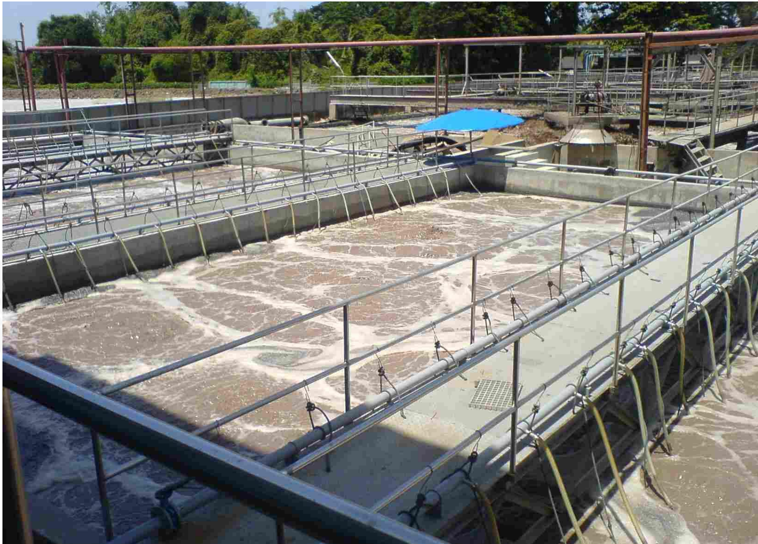
Aeration basin for activated sludge process
