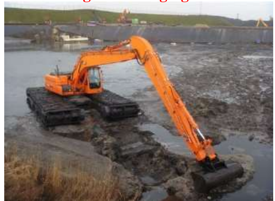
De-silting and Dredging of river
