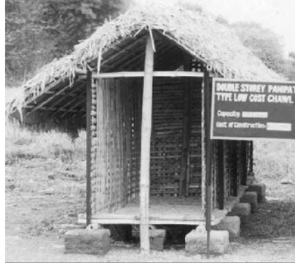
Fig. 16: Low cost bottom ventilated structure
