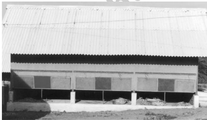
Fig. 15: Top and bottom ventilated storage structure
