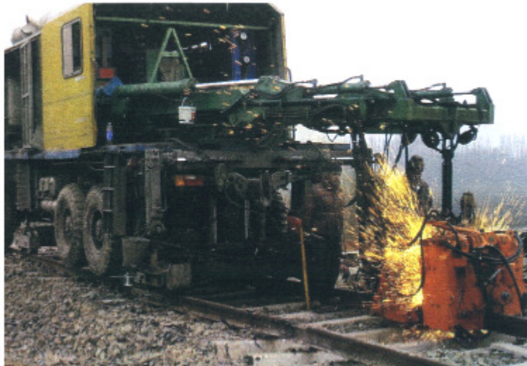
Flash-Butt Rail Welding with mobile Unite in India
