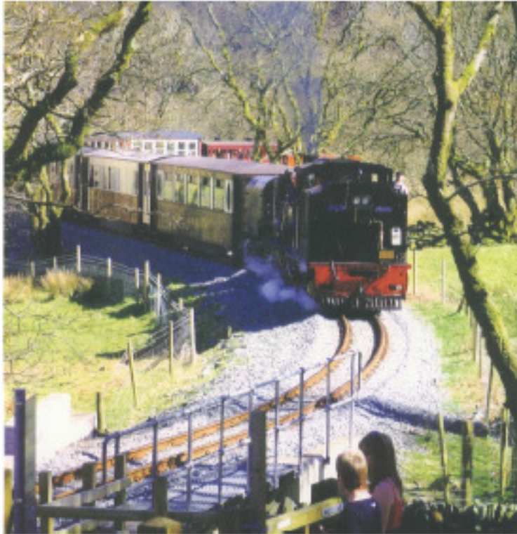
WELSH HIGHLAND RAILWAY, 2014, on a modern completely new rebuild 2 ft NG Rail Road, UK, with a well ballasted Rail Track and Steel Sleepers
