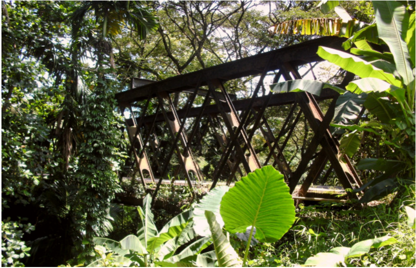
NG Railway Bridge left near Opanayake
