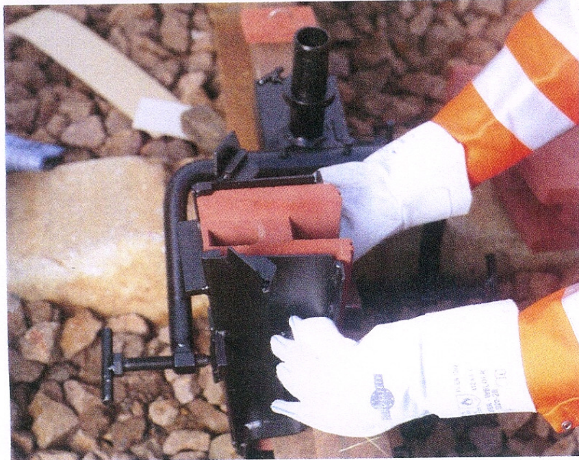
Fig. 20-6: Adjusting and positioning the mould
