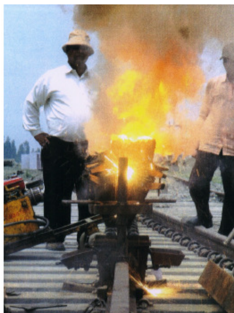
Alumino-Thermic Thermit-Welding on Rail Track in India
