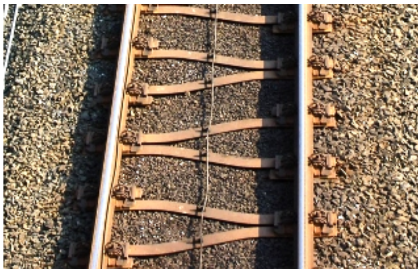
ThyssenKrupp Y-Steel Sleepers; 160 kmph CWR Line, Germany
