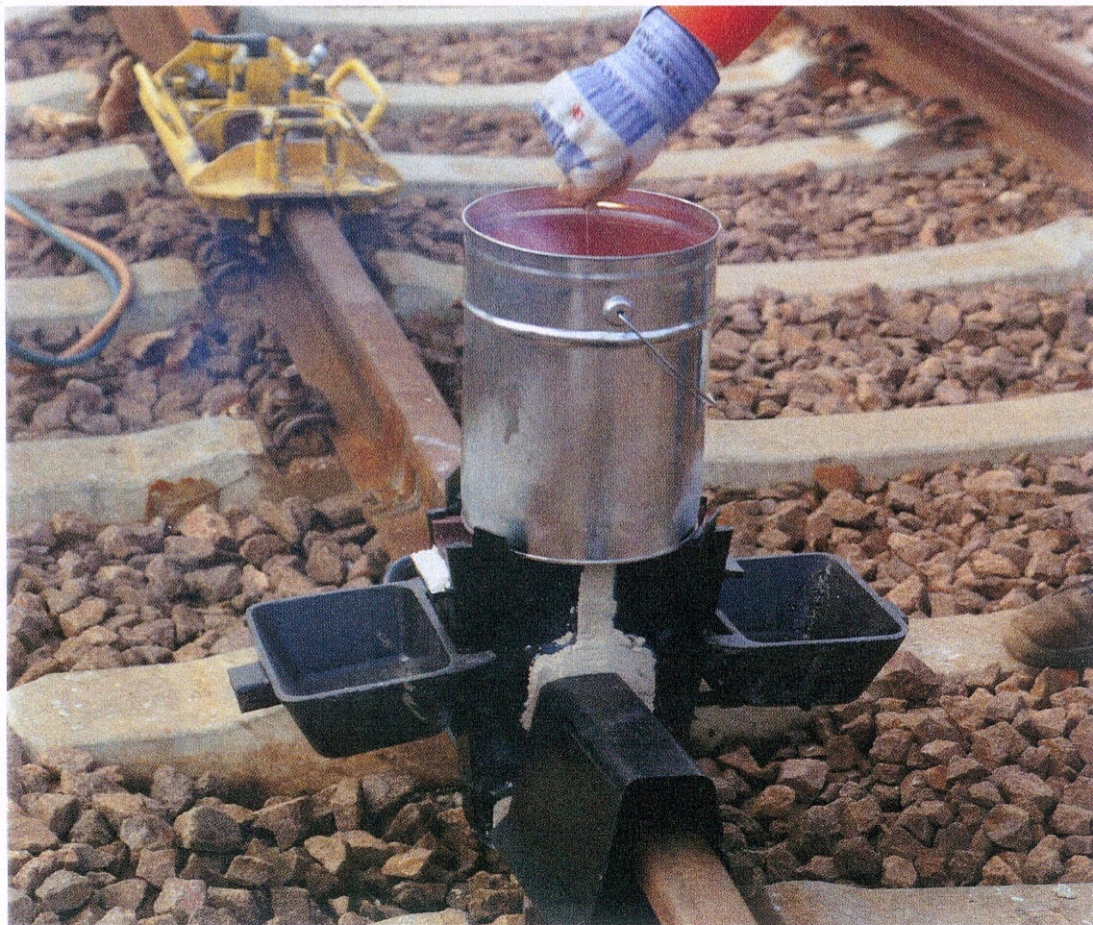
Fig. 20-9: Igniting the welding portion
