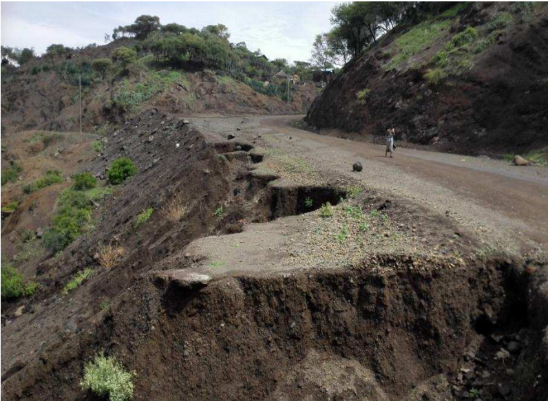
Failure due to thick layer placed compacted
