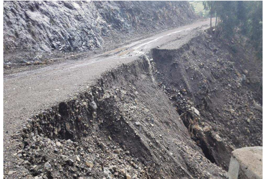
Failure due to thick layer placed compacted
