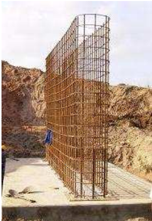
Reinforcement for a bridge pier
