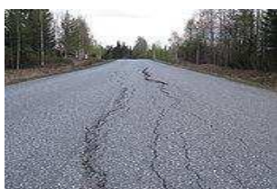
Pavement Cracks
