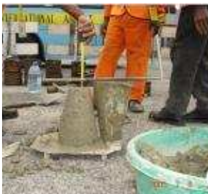
Measuring the Slump
