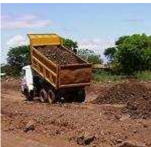
Dumping Gravel materials
