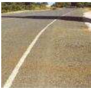
Typical Double Seal
