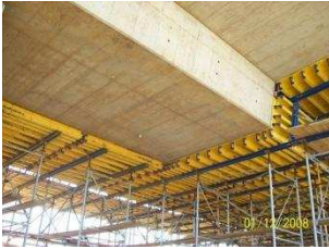
Proper formwork improves Workmanship
