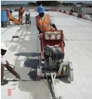
Un-reinforced concrete structure
