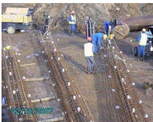
Reinforcement for cast in-situ piles
