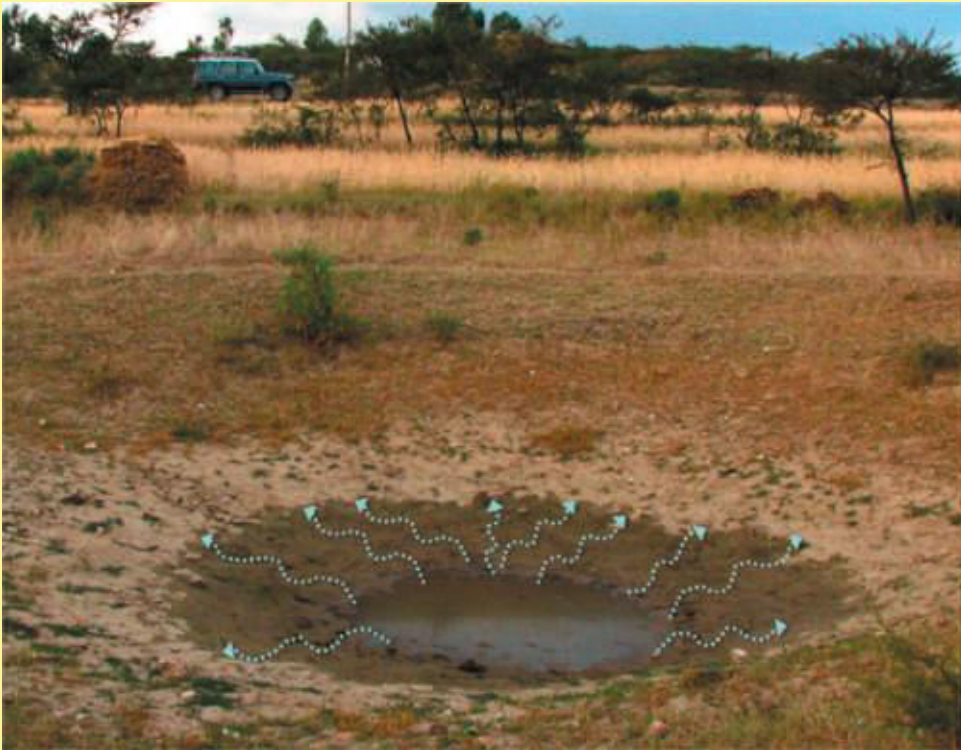
Surface runoff collection basin
