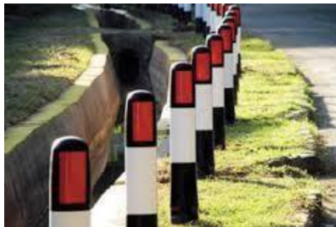
FIG.18 HAZARD MARKERS (a)
