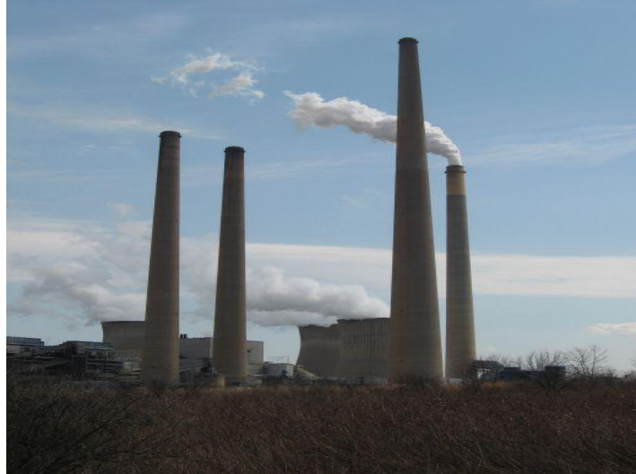
SMOKE STACK (CHIMNEY)
