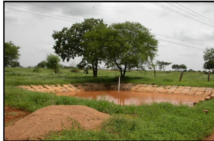
Fig. 15.2 Farm Pond Lined with Kadapa Slabs
