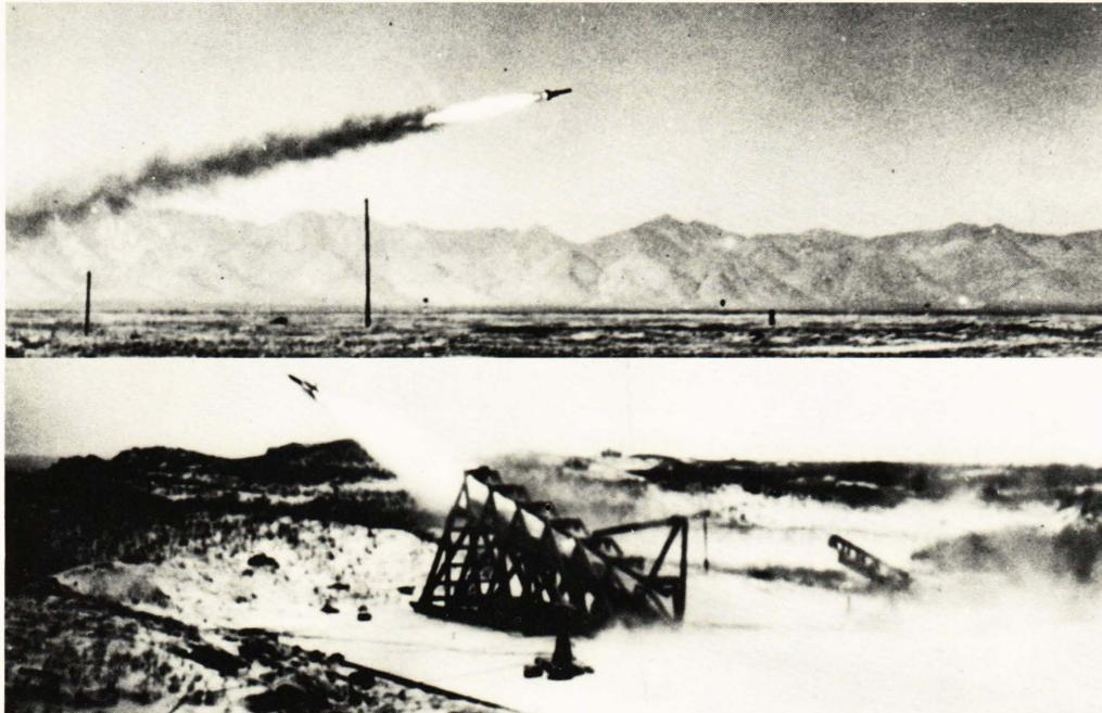
THE BUMBLEBEE—Here is a model of the Navy's new ram jet engine called "The Bumblebee," taking off from a launching platform (bottom photo). The model in flight (upper photo) is capable of supersonic speeds up to 1,500 miles per hour at high altitudes.
