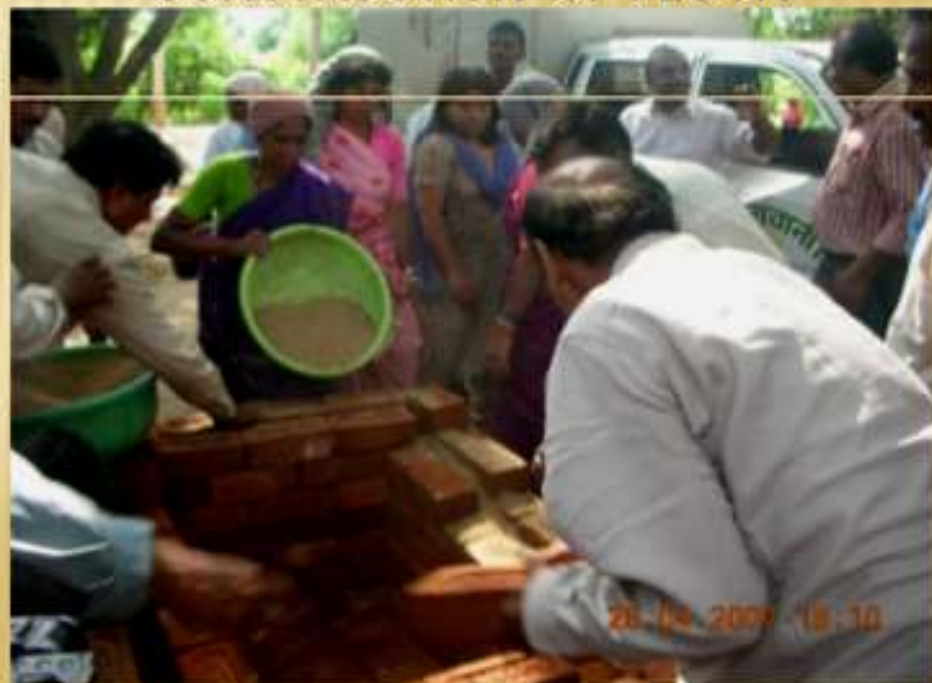
CAVITY FILLED WITH SAND
