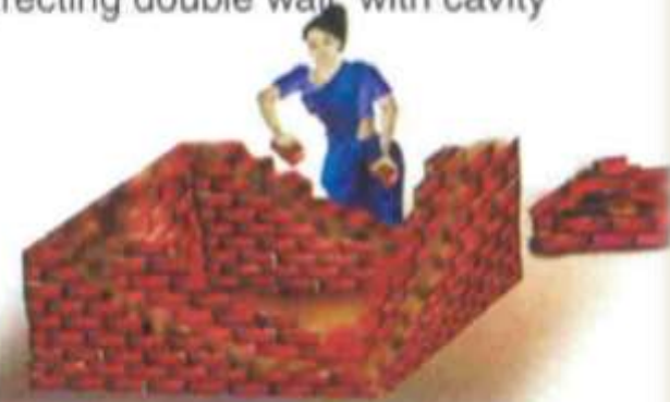
Erecting double wall with cavity
