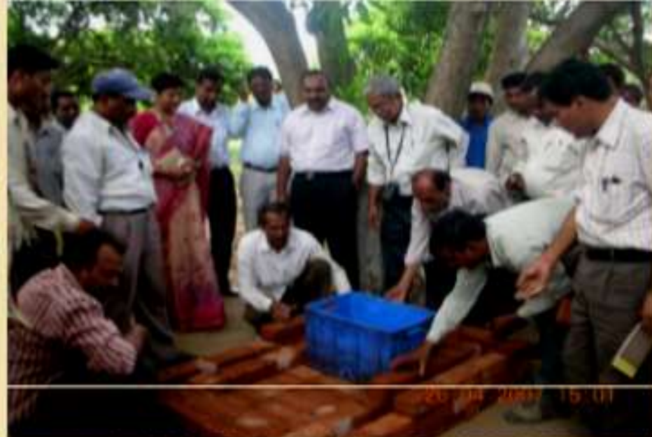
CONSTRUCTION OF FLOOR
