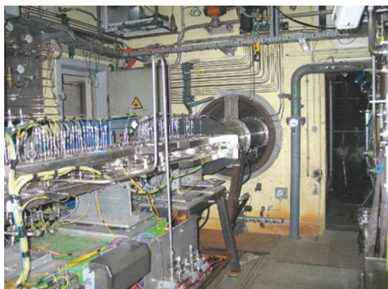
Figure 37 - View of the test setup in the ATD 5 test cell
