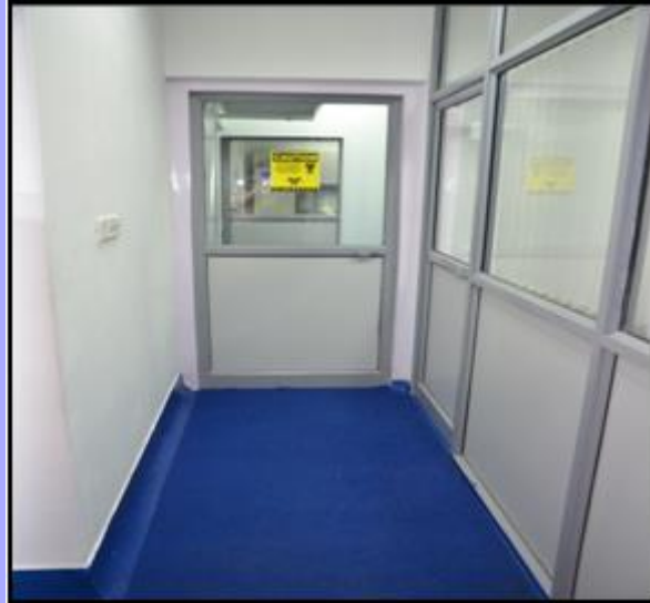
Fig. 22.7 Doors for access control
