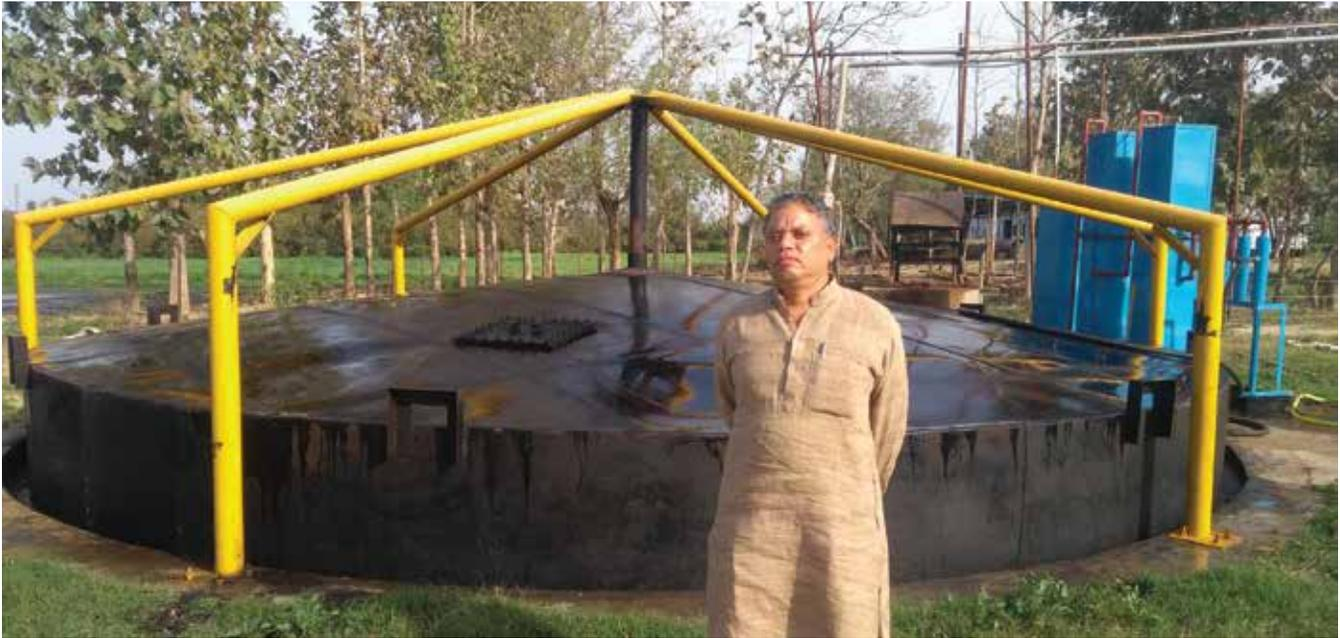
*Biogas Power Generation (Off-grid) Project at site of beneficiary Sri Ramji Gupta, Vill- Bhatauli, Post- Rura, Dist- Kanpur Dihat (Biogas Capacity 140 m<sup>3</sup> / 16 KW)*
