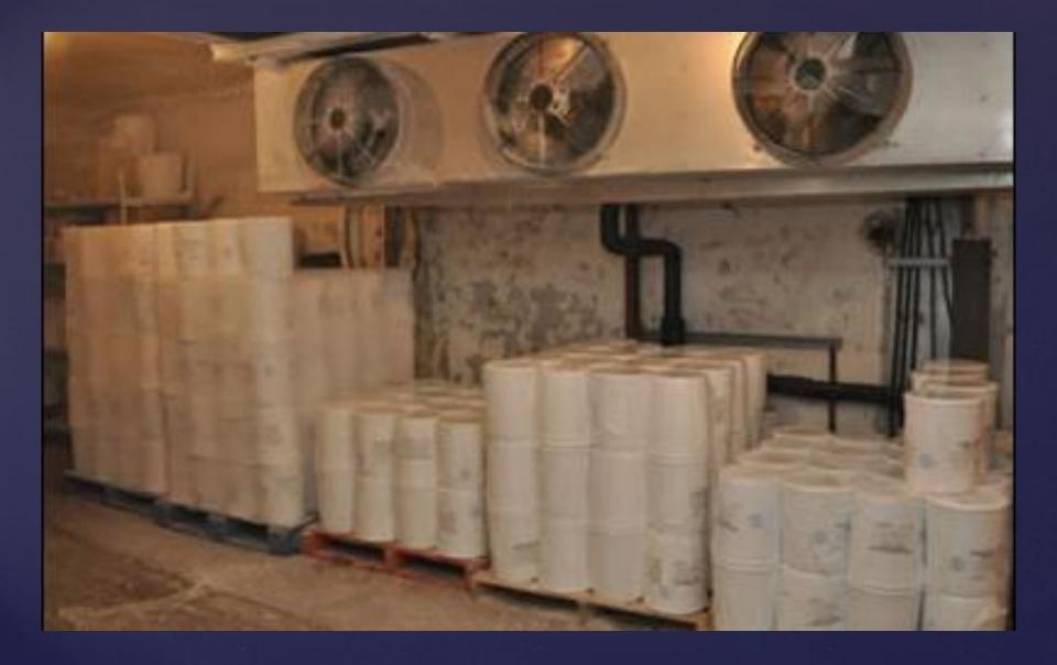
**iii)** Forced air type hardening room: The expansion coils are in the form of a compact unit utilizing fins to assist in the conductance of heat from the air to the coils. A fan placed directly behind the expansion coil unit, draws the air from the hardening room and blows it over the expansion coils and back into the room.
