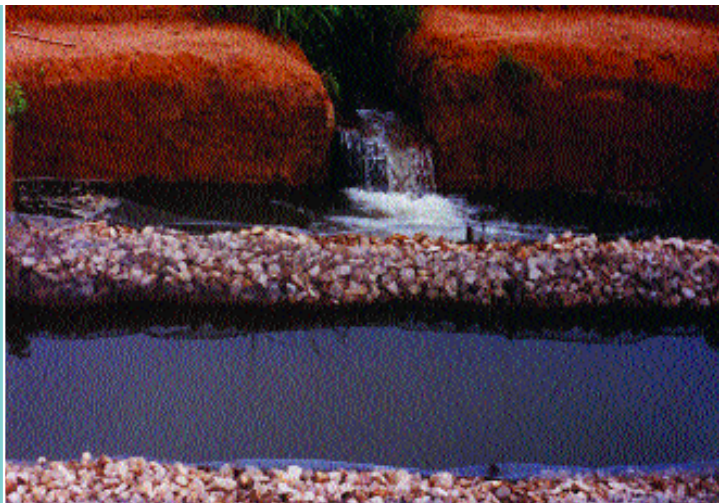
Figure 51 Simple gravel filters on the water intake system help to minimize the predators in freshwater prawn ponds (Peru)
