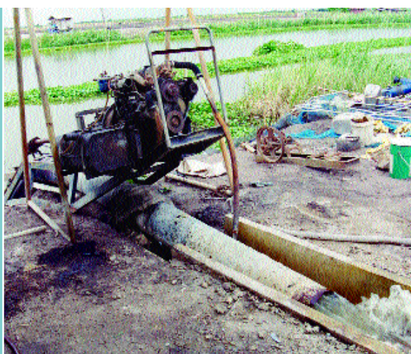
Figure 9 Pumps can be powered by old diesel bus engines (Thailand)
