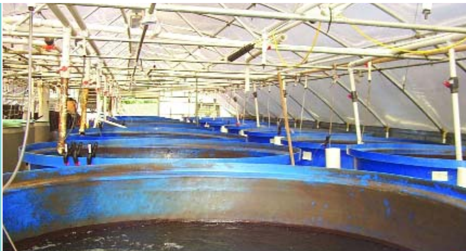
Figure 38 Overhead air and water distribution systems are used to supply these indoor nursery tanks (USA)
