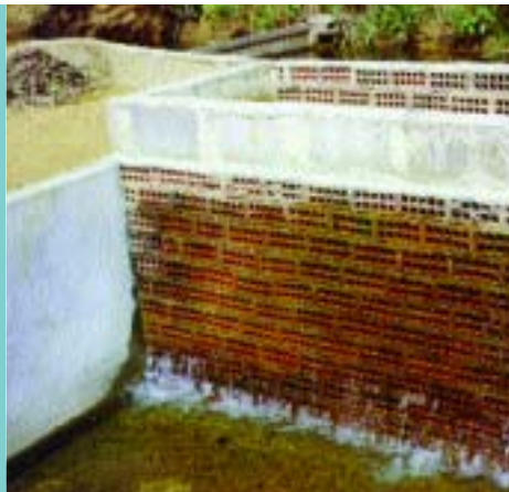
Figure 79 A simple gravel filter on a farm supply system helps to exclude predators (Brazil)
