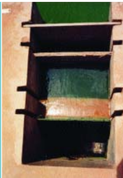
Figure 56 The outlet structure, sometimes known as a 'monk', can be used to control the level of the water as well as to screen the water to prevent the loss of freshwater prawns (Brazil)
