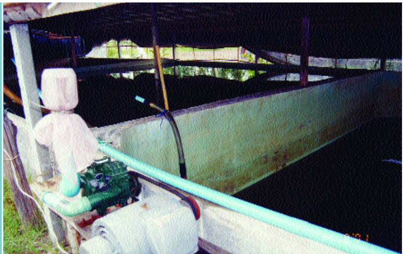
Figure 25 Tanks for storing hypersaline water and freshwater, and for mixing purposes at an inland hatchery in Thailand; note the roof and side covers for excluding aerial pollution and controlling temperature
