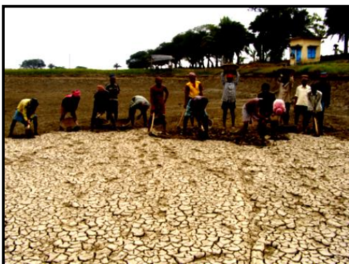
Top soil removal
