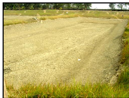
Pond bottom after top soil removal
