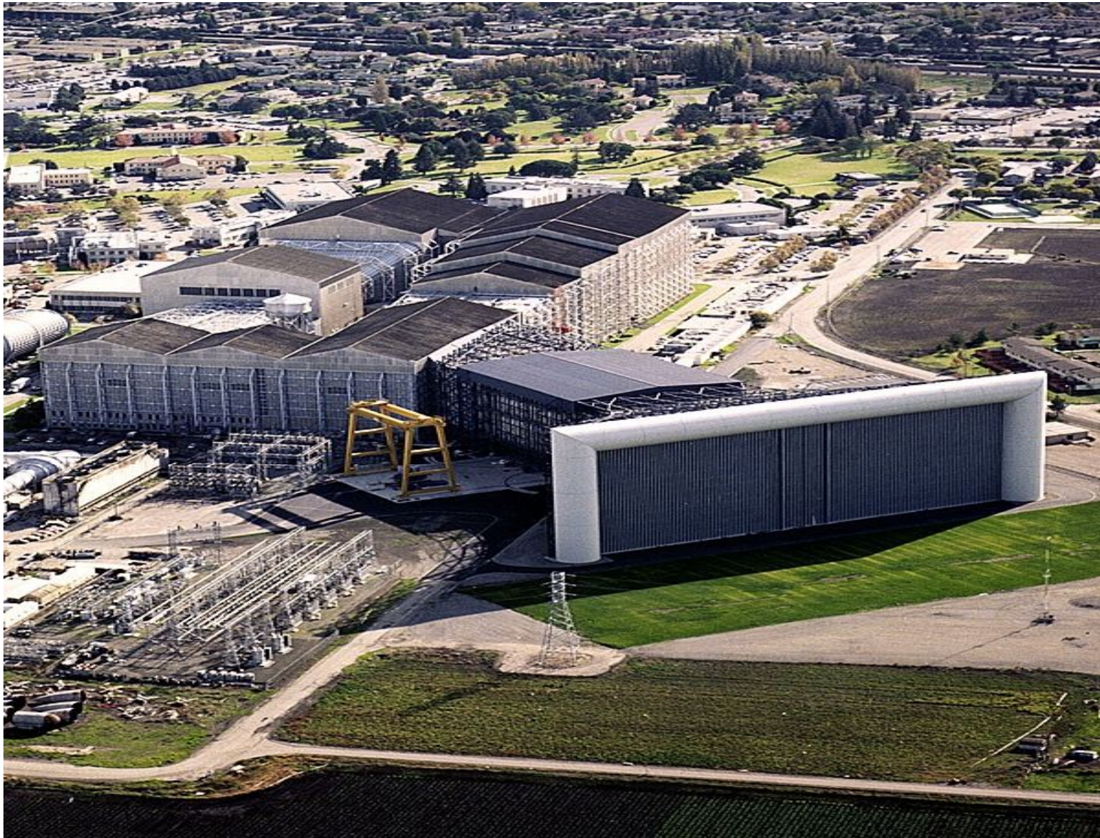
NASA AMES RESEARCH CENTER'S 80 FT X 120 FT OPEN-CIRCUIT "SUCKDOWN" TUNNEL, WITH SIX FAN AT EXIT
