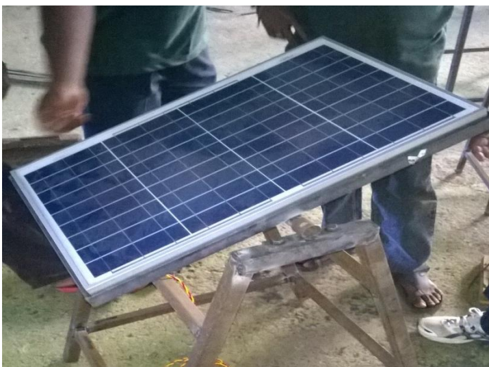
Figure 3.5. Shows the installation of PV panel
