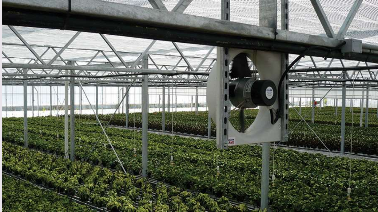
Horizontal air flow (HAF) cooling
