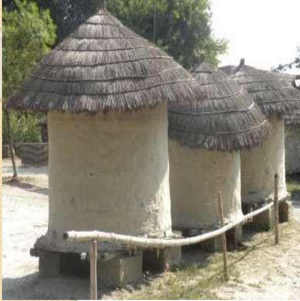
Mud bin structure
