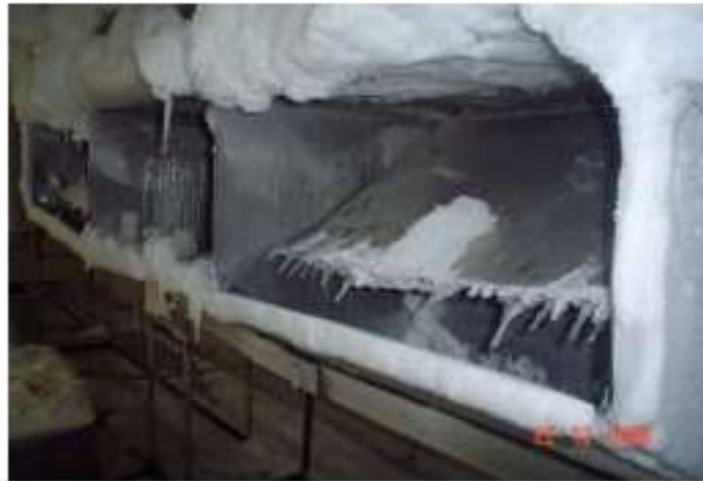
Fig 2. Frost on a duct of a refrigerating unit in a cold store
