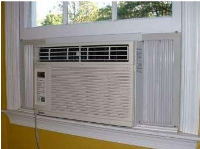
Window Air Conditioning
