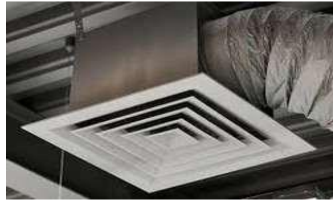
Centralised Air Conditioning
