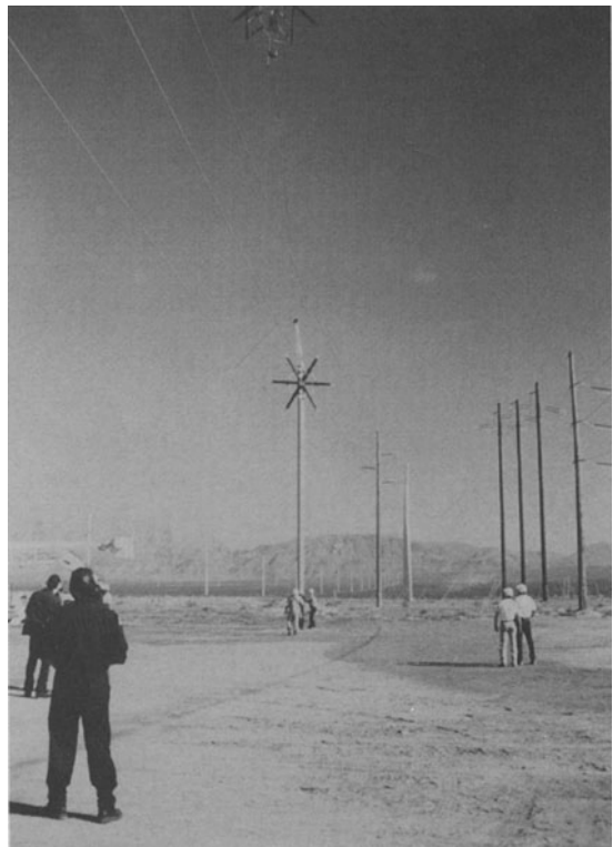
Fig. 43.5 Installing lightweight composite utility poles by helicopter. (Courtesy of Amoco Chemical Co.)
