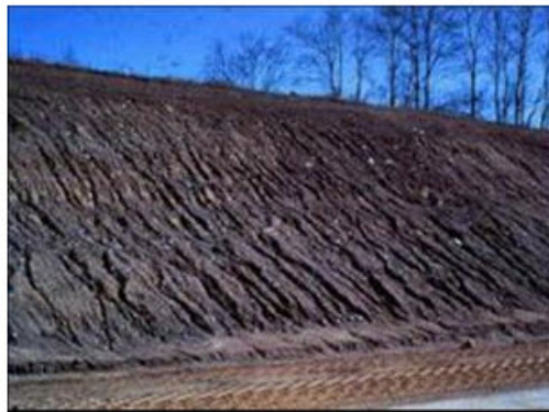
Fig. 3.3. Rill erosion. (Source: http://www.kalkaskacounty.net )
