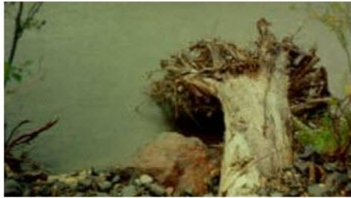
Fig. 12.8. Rootwads Armor to Protect the River Bank in-stream Structures.
