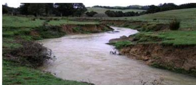
Fig. 12.1. Stream Bank Erosion Showing Slump and Meandering.
