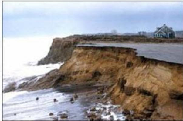
Fig. 3.6. Sea-shore/ coastal erosion.
