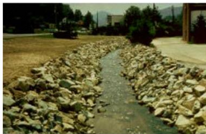
Fig. 12.5. Riprap for Protection of River Bank.
