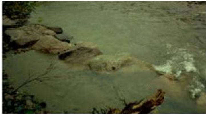
Fig. 12.9. Rock Vanes for Protection of Stream Bank.
